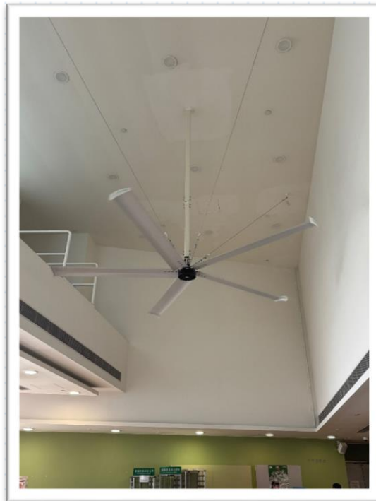
Figure 5-2: Low-speed-high-volume fan in the canteen
