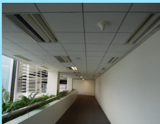
Figure 5-1: De-lamping in common area
