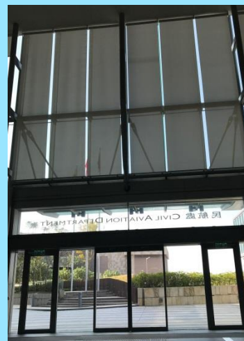
Figure 5-5: Motorized blinds at the atrium of CAD Headquarters shield sunlight effectively
