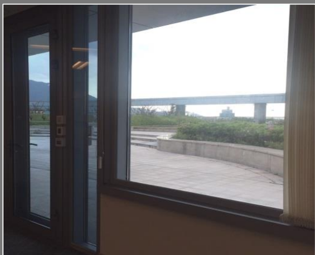
Figure 5-5: An example of showing the effect of solar films shielding the office area from sunlight effectively (glass panel on the right without solar film installed)
