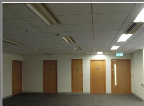
Figure 5-1: De-lamping in common area
