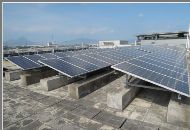
Figure 5-6: Photovoltaic panels on the rooftop of CAD Headquarters
