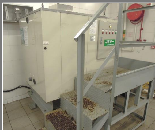
Figure 5-12: The food waste decomposition system in CAD Headquarters
