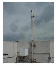
Figure 2-5: Outdoor noise monitoring terminal
