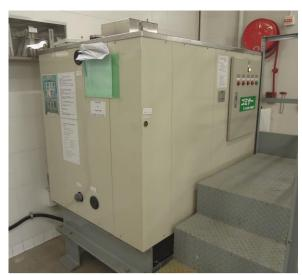
Figure 5-7: The food waste decomposition system in CAD Headquarters
