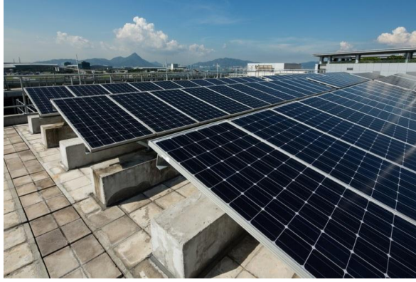
Figure 5-3: Approximate 130 m 2 of Photovoltaic Panels
