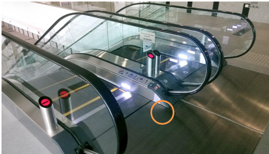
Figure 5-9: Escalator with services-on-demand sensor
