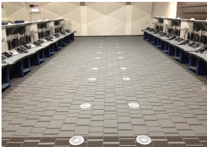
Figure 5-6: Separation of air-conditioning for equipment and occupant
