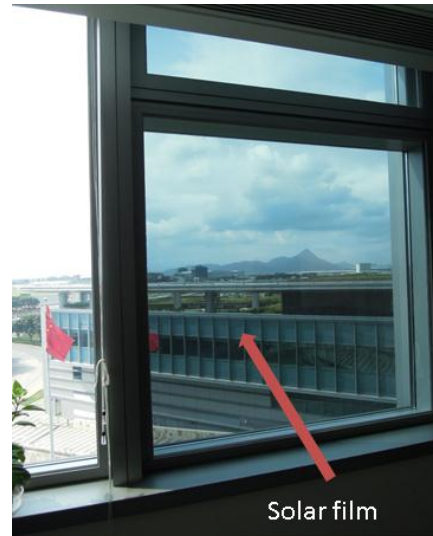
Figure 5-12: Solar films are installed in strategic locations to reduce sunlight and heat
