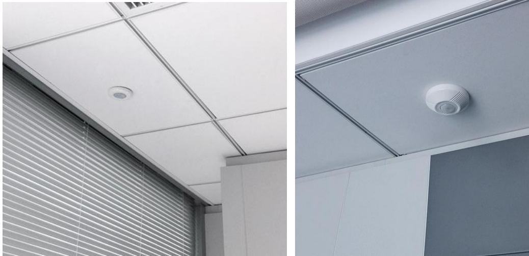
Figure 5-5 : (Left) Daylight Sensor and (Right) Occupancy Sensor
