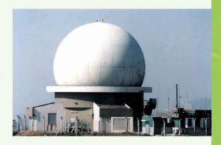
tube design and 3 MW peak transmission power by a new fully solid-state radar with 24 kW peak transmission power, but with the same radar coverage, at the end of 2003.
