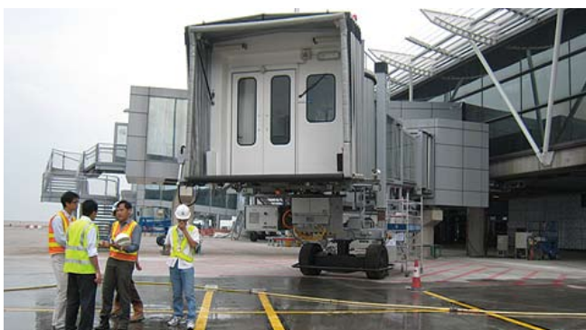
本部同事在北客運廊進行視察。 Divisional colleagues conducting a site inspection of the North Satellite Concourse.
