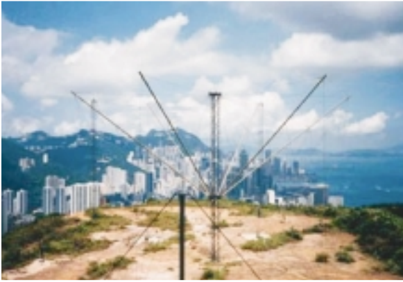
◁ 民航處於畢拿山的高頻螺旋錐形接收天線 CAD HF Spiracone Receiving Antenna at Mount Butler
