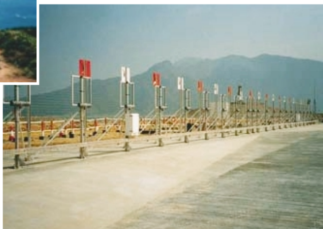
^ 儀表著陸系統(航向信標天線) Instrument Landing System (Localiser)
