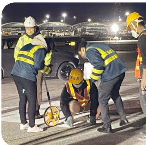
Colleagues from the Airport Standards Division conduct compliance check on the new runway designation marking.
