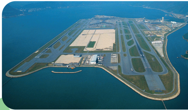
On 18 May 1999, the North Runway of the HKIA that catered for the new generation of ultra large aircraft opened for operations. (Photo source: Airport Authority Hong Kong)
