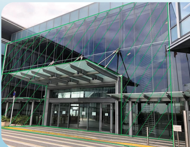
Solar control window films applied to the curtain wall fenestration at the main entrance of the CAD HQs reduce the heat load from the sun transferred to the central air conditioning system.
