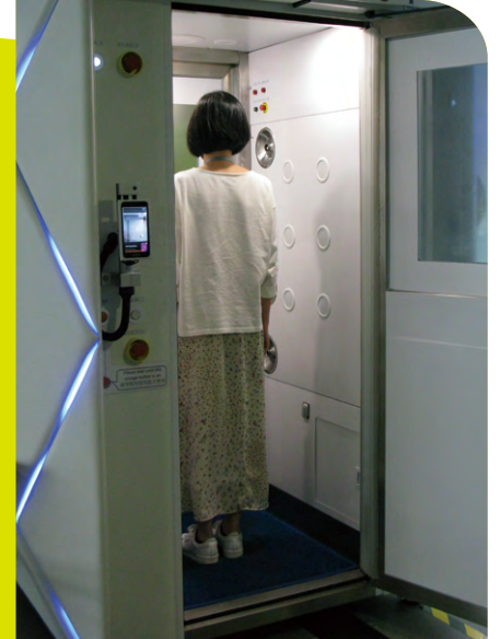
Smart body disinfection chamber is installed at the Air Traffic Control Building. 航空交通管制大樓地下安裝智能消毒系統。
