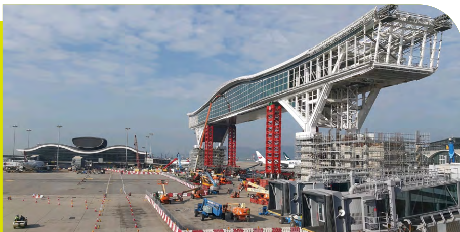
The main structure of the Sky Bridge erected at its final position between Terminal 1 and the NSC. 天際走廊主結構豎立於其最終位置，位於一號客運大樓及北衛星客運廊之間。
