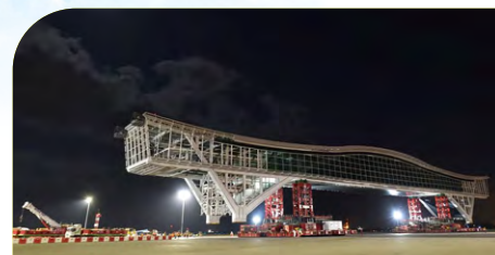
To minimise disruption to airport operation, the delivery of the Sky Bridge commenced at the early hours of 9 January. 為減少對機場運作的影響，天際走廊的運送過程於1月9日凌晨展開。
