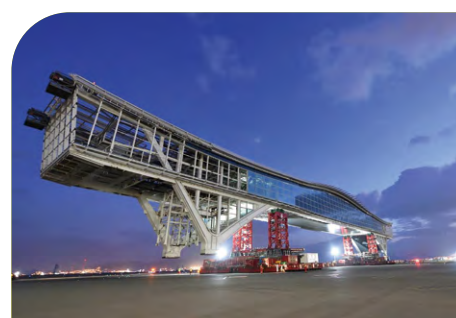
The main structure of the Sky Bridge was close to being delivered to its designated position at the break of dawn. 天際走廊主結構於清晨時分逐漸運抵指定位置。
