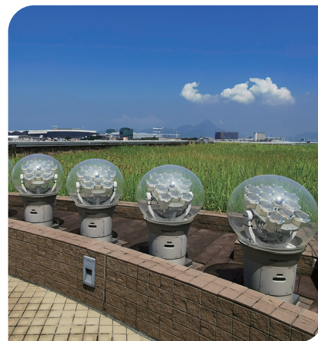
The solar tracking optical fiber lighting system installed at the CAD Headquarters.
