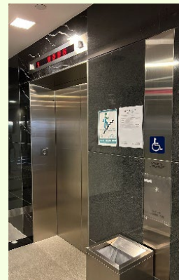
Figure 5-1: Lifts programming to reduce wastage during non-peak office hours
