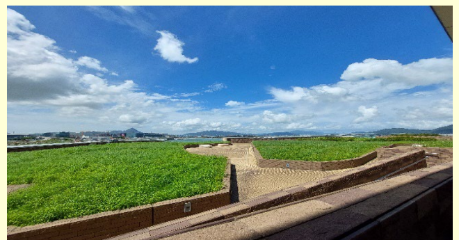
Figure 5-6: Green roof helps lower temperature on the top floor
