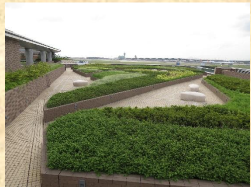
Figure 5-6: Green roof helps lower temperature on the top floor
