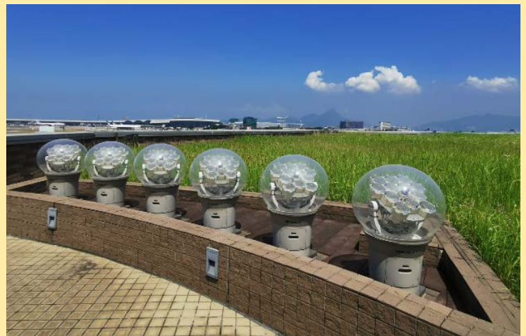
Figure 5-5: Green roof helps lower temperature on the top floor
