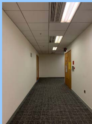
Figure 5-2: Replacing obsolete and less energy efficient tubes with T5 tubes
