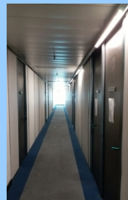
Figure 5-2: Replacing obsolete and less energy efficient tubes with T5 tubes
