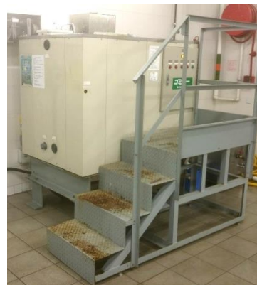
Figure 5-12: The food waste decomposition system in CAD Headquarters
