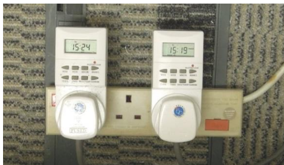
Figure 5-4: energy-saving timer devices connected to photocopiers
