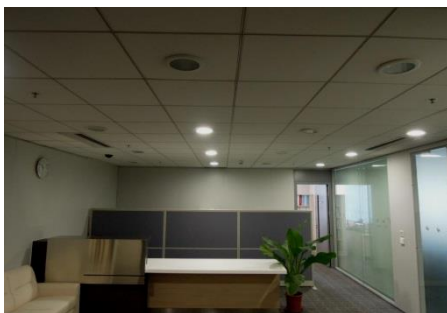
Figure 5-1: De-lamping in common area
