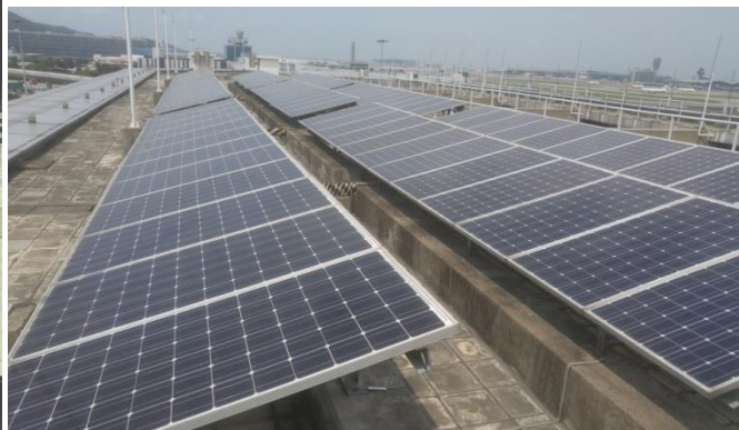
Figure 5-6: Photovoltaic panels on the rooftop of CAD Headquarters
