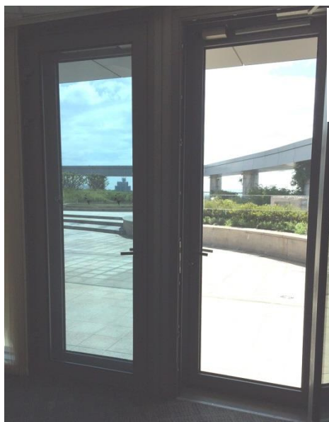
Figure 5-5: An example of solar films shielding the office area from sunlight effectively (glass panel on the left with solar film installed)
