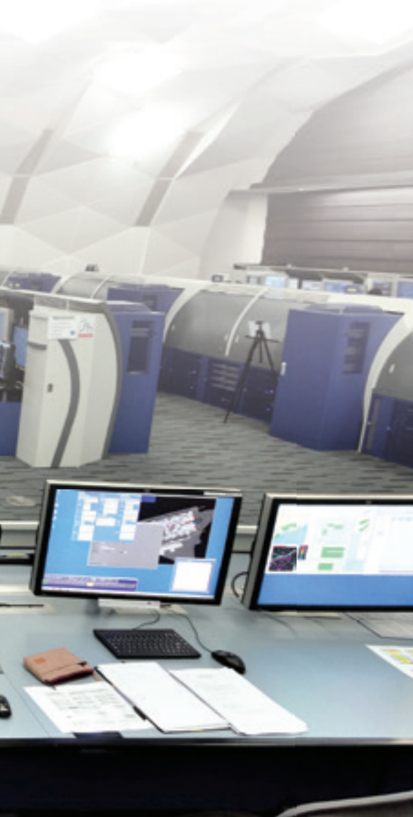
東空管中心的新空管系統投入運作。 The new ATC systems were commissioned at the E-ATCC for operational use.
