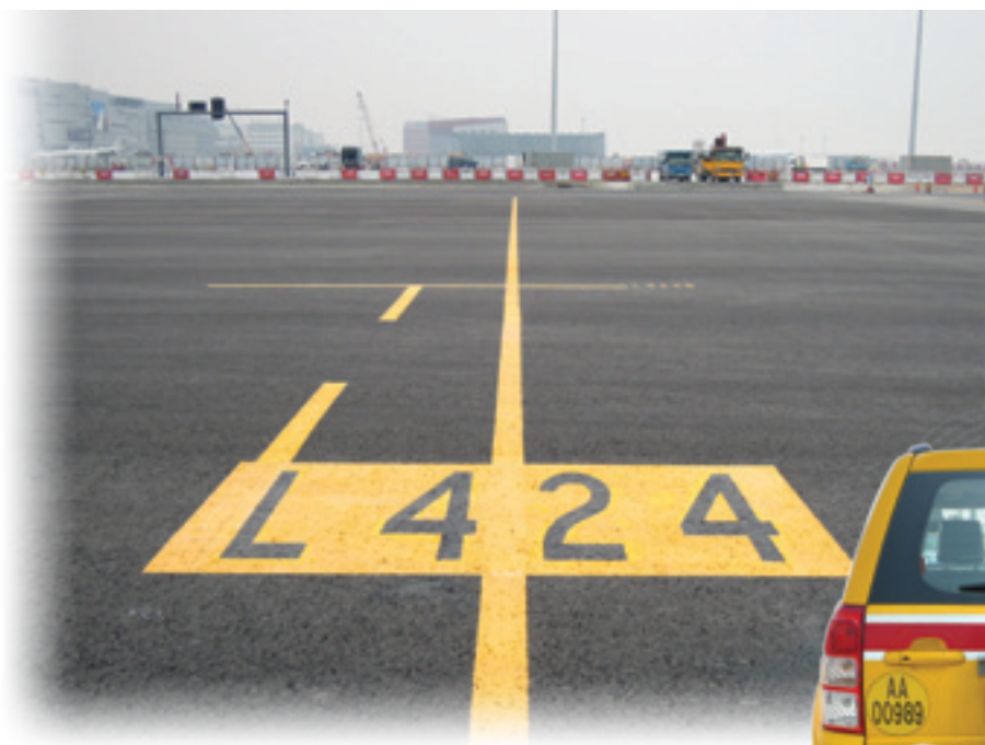
機管局按照國際民航組織的要求，在新停機坪上設置停機位標誌。 Aircraft stand marking in compliance with ICAO requirement provided by AAHK on the new parking apron.
