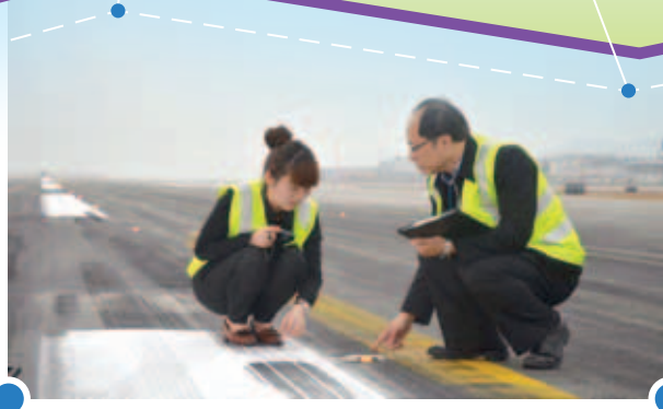
機場安全標準部人員巡查北跑道的飛行區地面燈號系統。 APSD officers inspecting the airfield ground lighting system on the North Runway.
