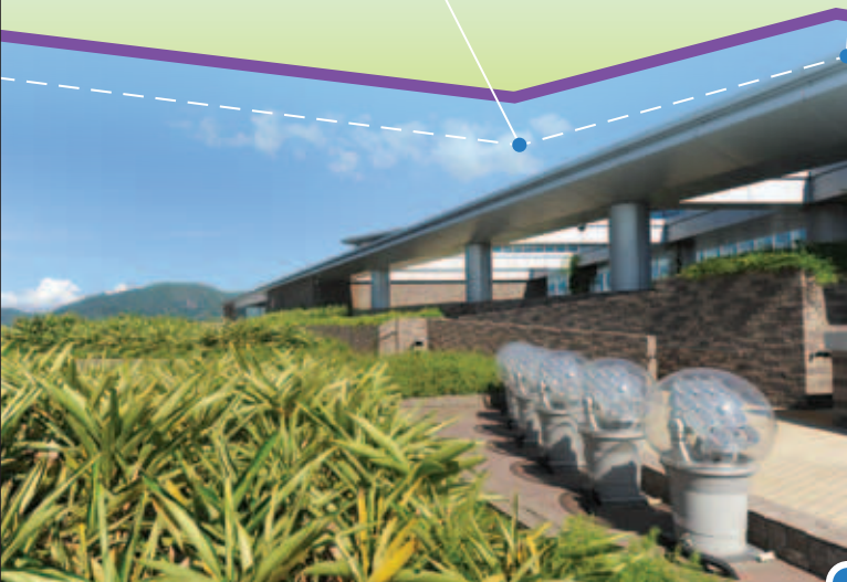
天台花園裝設了光導太陽光收集裝置。 Solar lighting collectors with fibre optic solar tracking are installed at the roof garden.
