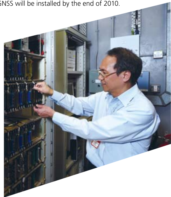
同事在儀表著陸系統儀器室內工作。 Staff works in the Instrument Landing System equipment room.
