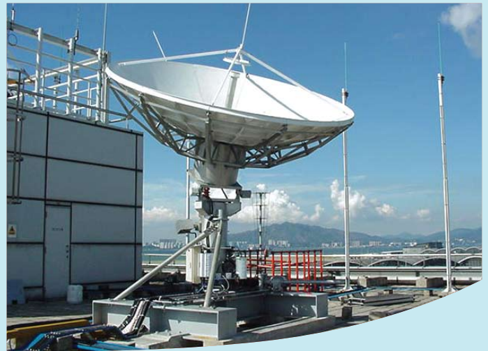
設於航空交通管制大樓天臺的衛星天線。 Satellite antenna on the roof of Air Traffic Control Complex.
