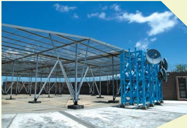
位於小磨刀多普勒甚高頻全向無線電信標及測距儀。 Doppler Very High Frequency Omni-directional Radio Range and Distance Measuring Equipment (DVOR/DME) System at Siu Mo To.
