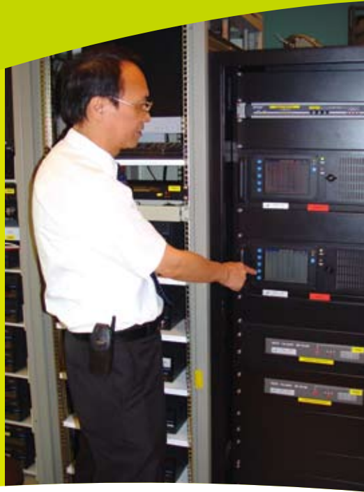
▲ 電子工程師定期替雷達數據系統進行維修保養。 Electronics engineer carries out maintenance work regularly for the Radar Data Formatter.
