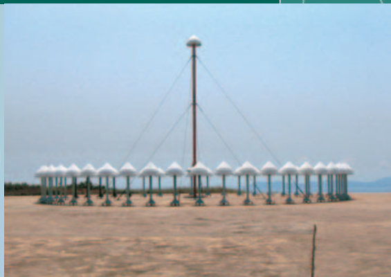
東龍島上的多普勒甚高頻全向無線電信標及測距儀。 The Doppler Very High Frequency Omni-directional Radio Range and Distance Measuring Equipment (DVOR/DME) on Tung Lung Island.
