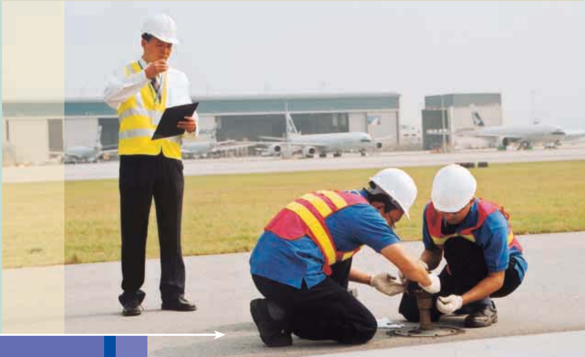
在民航處監察下，機場地面燈系統的質素不斷提升。 The Aerodrome Ground Lighting System continues to be upgraded under the inspection of CAD.
