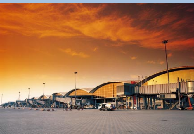
西北客運廊等機場新設施的安全及保安水平均受嚴密監管。 The safety and security standards of new airport facilities such as the Northwest Concourse are closely monitored.
