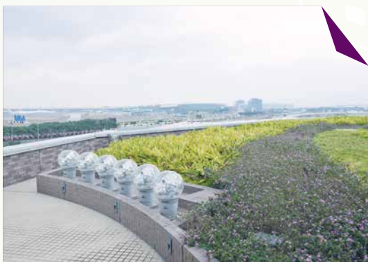
Solar lighting collectors with fibre optic solar tracking 光導太陽光收集裝置
