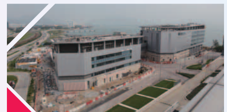
The construction of the New ATC Centre and the new CAD Headquarters has been making very good progress.
